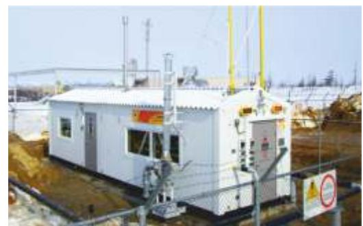
**Blocks of preparation, reduction and gas distributions units** are designed for the preparation of fuel gas for gas piston and gas turbine drives of compressor stations, power plants and other consumers.
