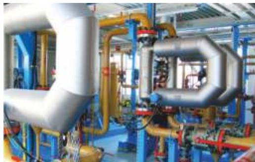
**Measurement Systems** are designed for automated quantity accounting crude, marketable oil or petroleum products indirect bulk or direct mass dynamic method according recommendations No. 69 of March 31, 2005, GOST R 8.595, MI 2825, GOST R 8.615, MI 2693.
