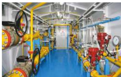
**Gas metering units** are designed to determine the quantity, quality parameters, automated metering of natural and associated petroleum gas.
