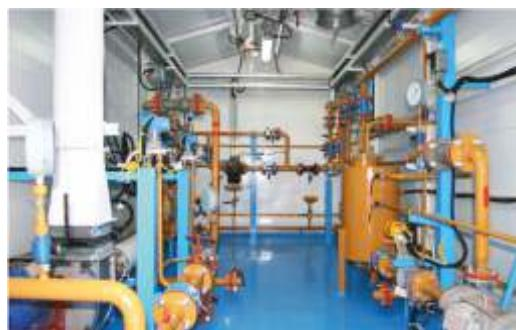
**Oil quality measurement units** designed for automatic definitions of physico-chemical indicators of oil quality according to GOST R 51858-2002, automatic and manual selection of oil samples for subsequent oil quality analysis.
