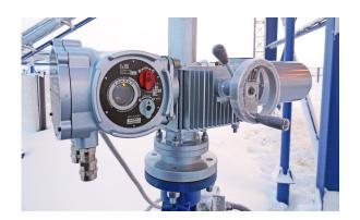
The explosion protection IP67 of the casing ensures the RemTEK operation under the water exposure and fully protects the drive against dust. The double sealing of the connection boxes protects the inside electronics against the environmental exposure.
