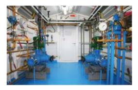
**Pumping stations** are designed for pumping oil, oil products, natural associated petroleum gas liquefied gas, gas condensate, water, chemical reagents and automated support set pressure at the outlet.
