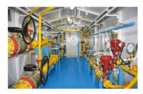
**Gas metering units** are designed to determine the quantity, quality parameters, automated metering of natural and associated petroleum gas.
